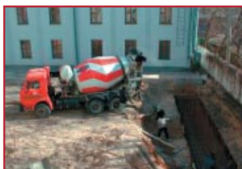
Following the arrival of spring, construction resumes.
